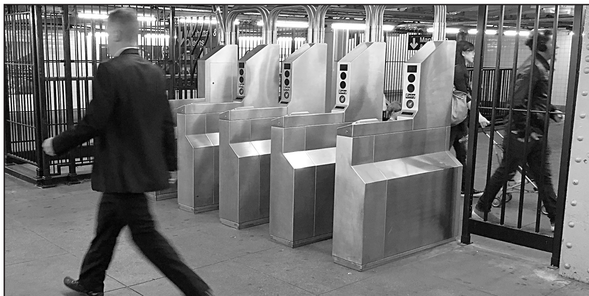
PB process includes dramatic improvements to the Seventh Ave. subway entrance.
